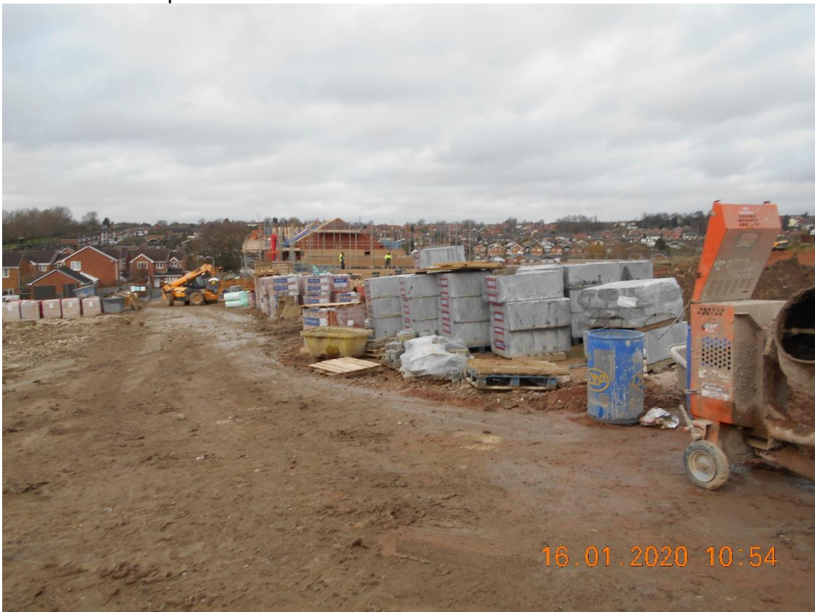
View from the top of Alton Drive towards the link section of Acorn Avenue
